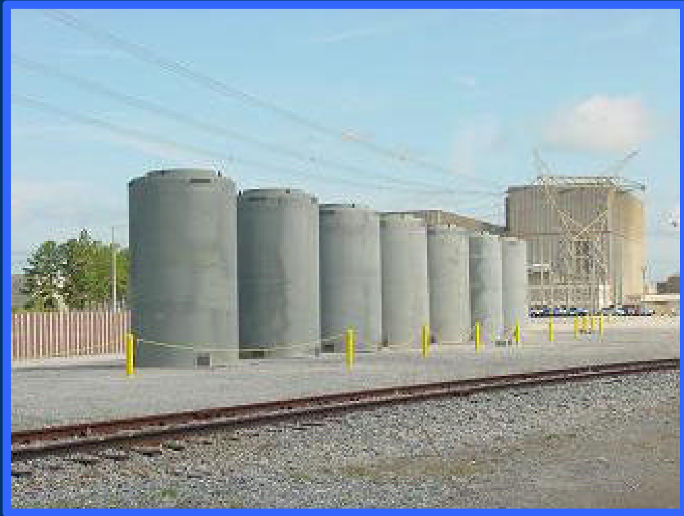
Vertical Dry Storage System at Reactor Site
