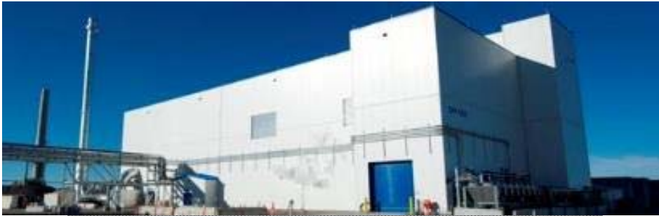
Integrated Waste Treatment Unit (ID)
