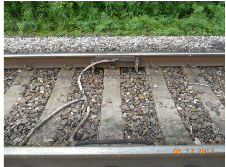
Closeup of Greaser Activators
