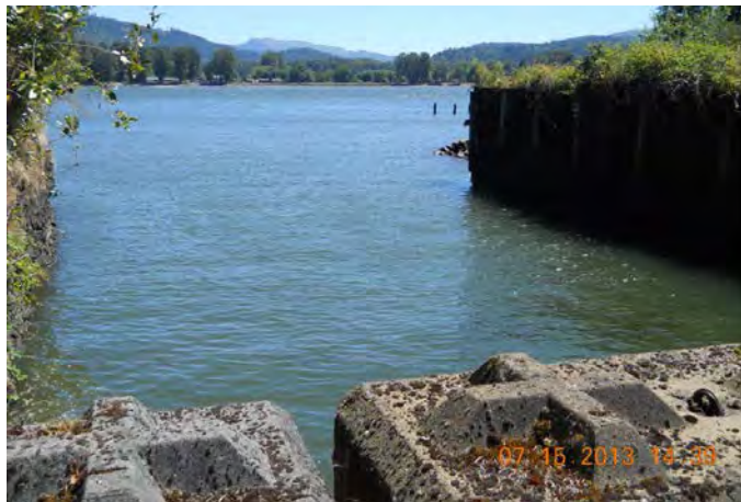
Barge Slip at Trojan
