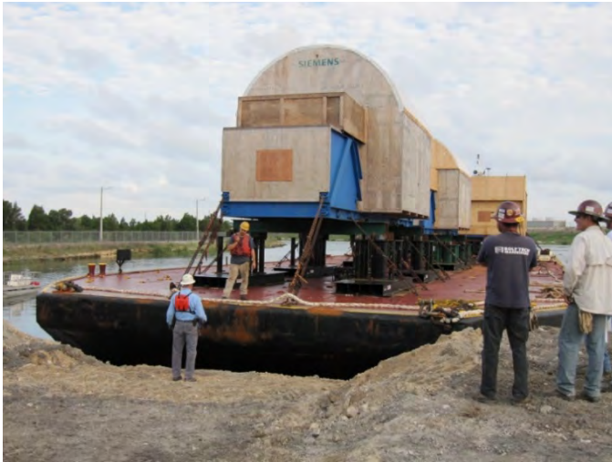
Turbine Component Unloading at Crystal River
