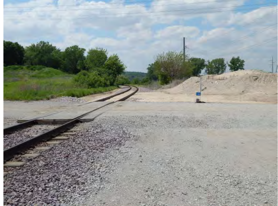
Cargill Rail Spur Looking Northwest
