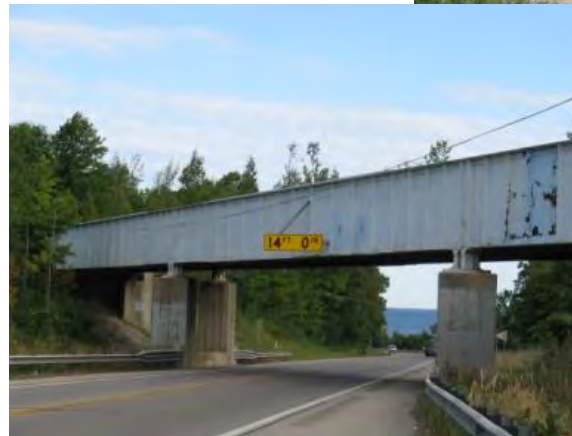
Low Overhead Bridge Near Big Rock Point
