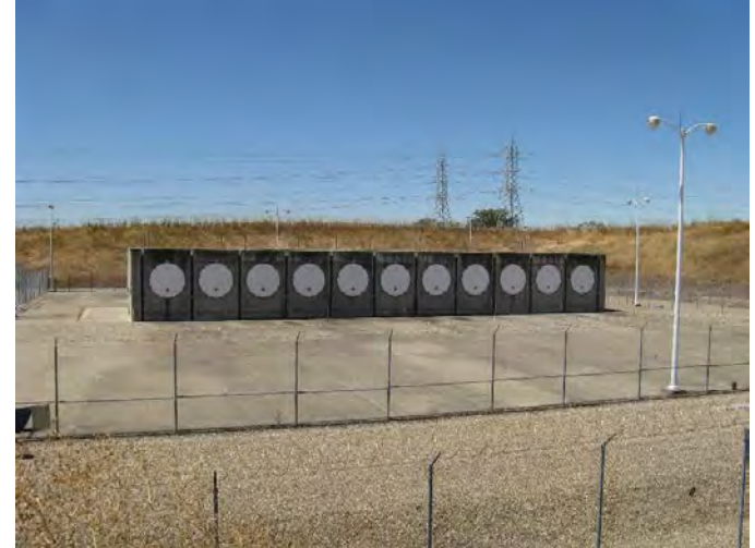
Horizontal Storage Modules (HSMs) Deployed at 5 Sites
