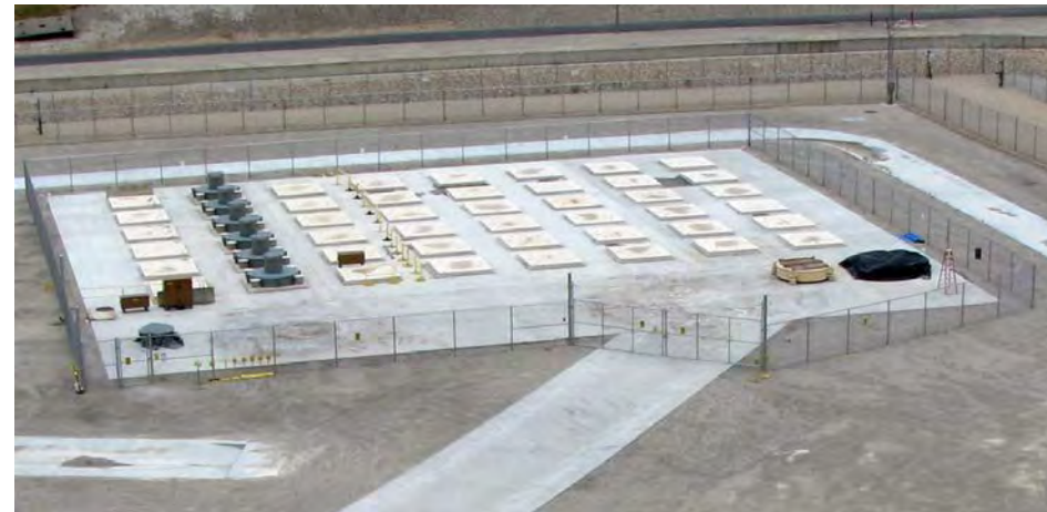
HI-STORM UMAX Underground Storage Modules
