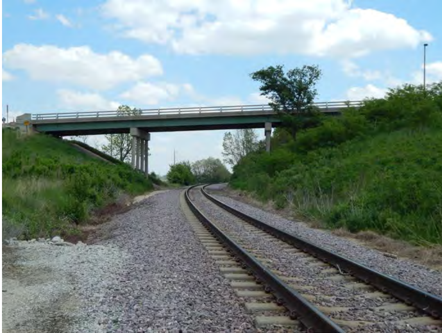
Cargill Rail Spur Looking Southeast
