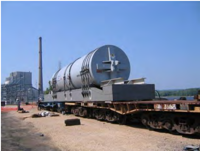
Reactor Pressure Vessel Shipping at La Crosse
