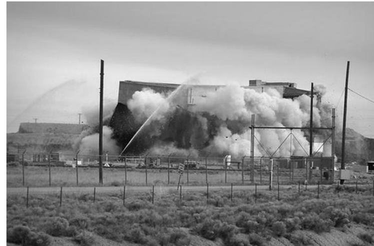
Workers demolish the Test Area North Hot Shop Complex, shown here.
