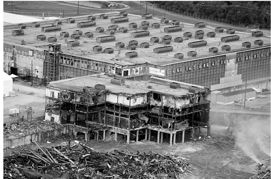
Workers begin demolishing the north end of the K-25 Building.
