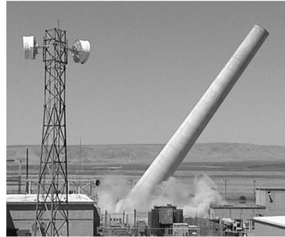
Workers safely demolished a 175-foot-high exhaust stack at the Hanford Site
