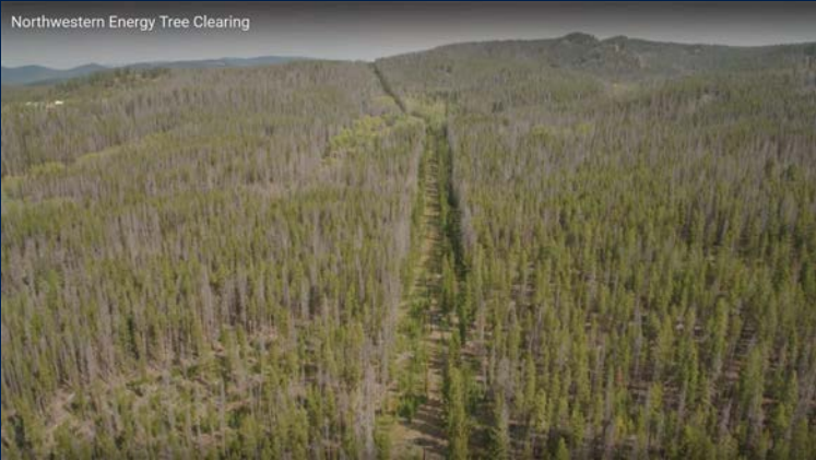
Northwestern Energy Tree Clearing
