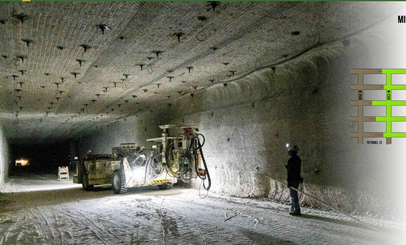
Above: Mining progress in the WIPP underground West Mains
