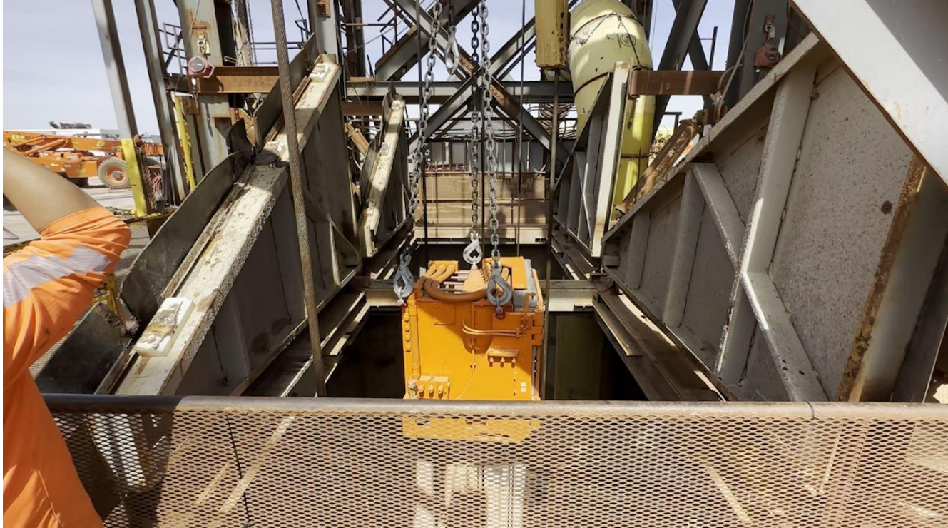
Lowering mining equipment down the new Utility Shaft
