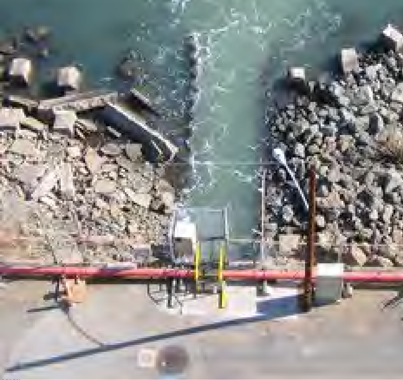
Return flow of heated water to San Francisco Bay from the Potrero Generating Station. (Source: Wikimedia Commons )
