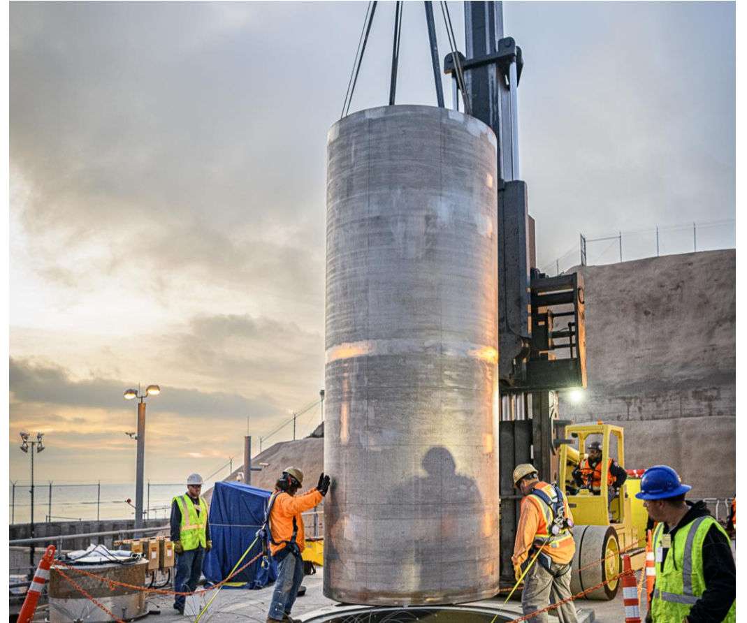
Test canister (no radiological material) installation at SONGS - https://www.songscommunity.com/decomm-digest/hope-for-the-new-year-factual-discussions-about-spent-nuclear-fuel -
